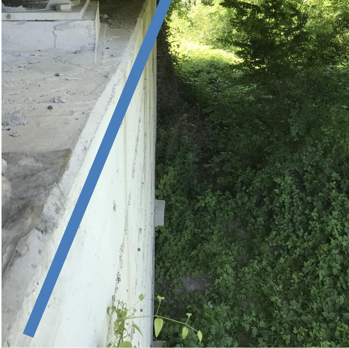
CANALA METALLICA STAFFATA A SPALLA PONTE – DX IDRAULICA
